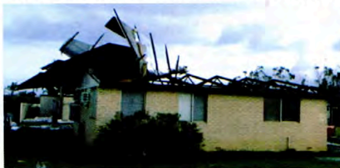
Figure 3.7 Roof blown away during cyclone
